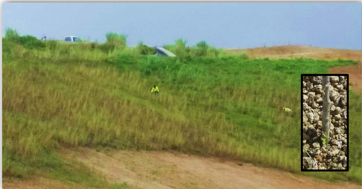
Figure 3 – Cover Maintenance, woody vegetation removal
