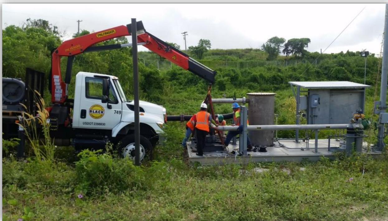
Figure 2 – Flare Station – Blower Replacement
